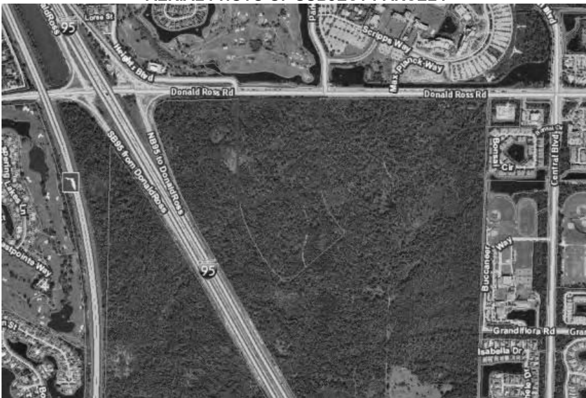
AERIAL PHOTO OF SUBJECT PARCEL II
